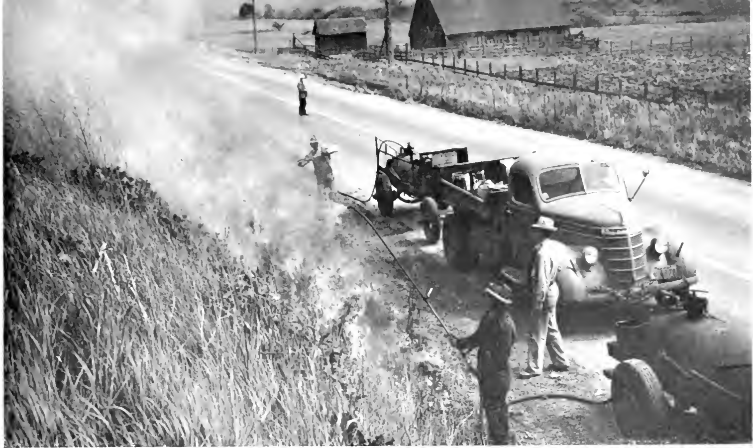
Burning oil-sprayed roadside growth. Fire is kept in control with water hose connections from truck tanks
